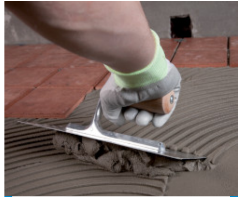
Application of Granirapid on terrace waterproofed with Mapelastic Zero
