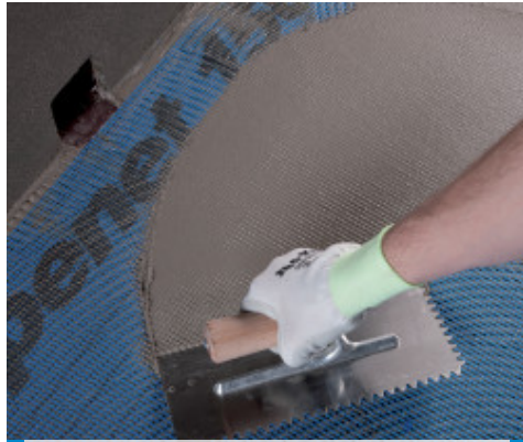
Application of Mapelastic Zero on Mapenet 150
